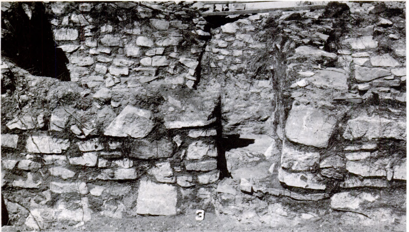
FIGURE 6 Masonry details and doorways in Room 3.
