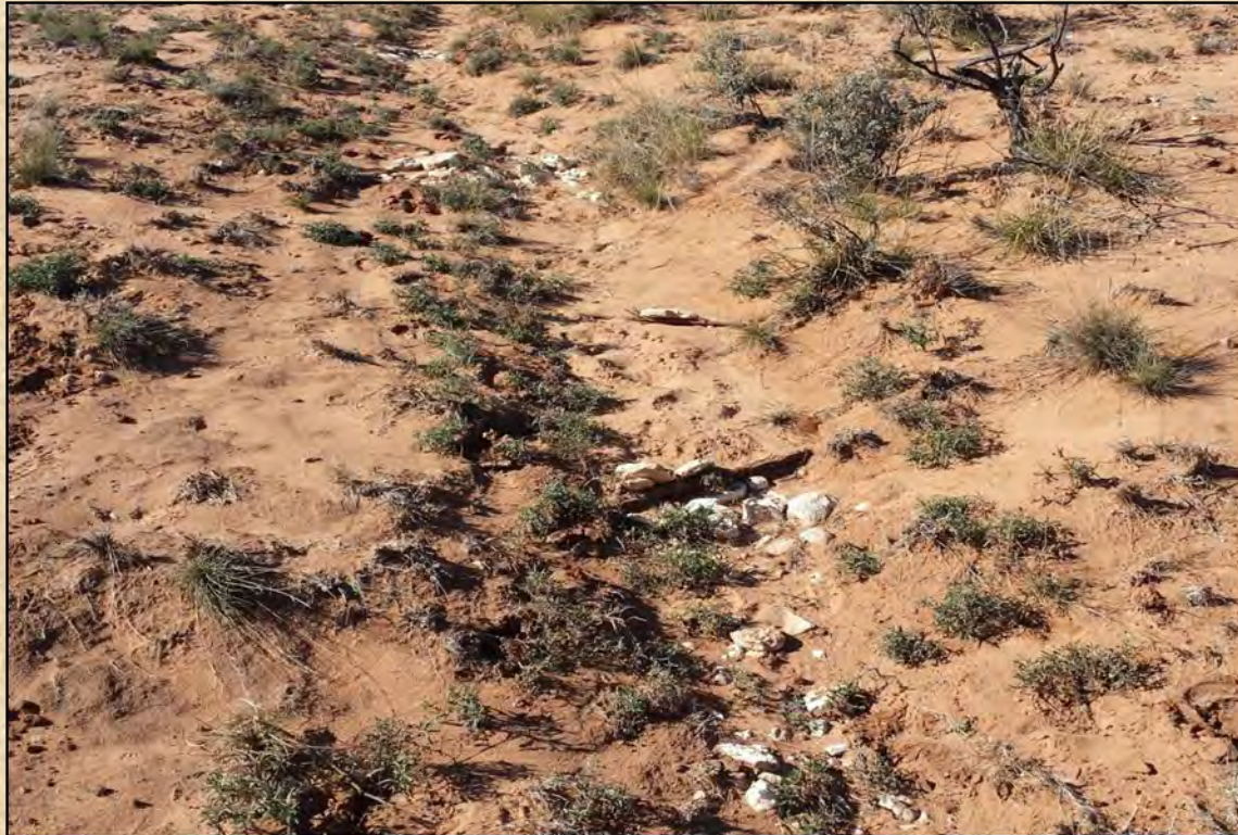
Check dams across the arroyo leading from the swale
