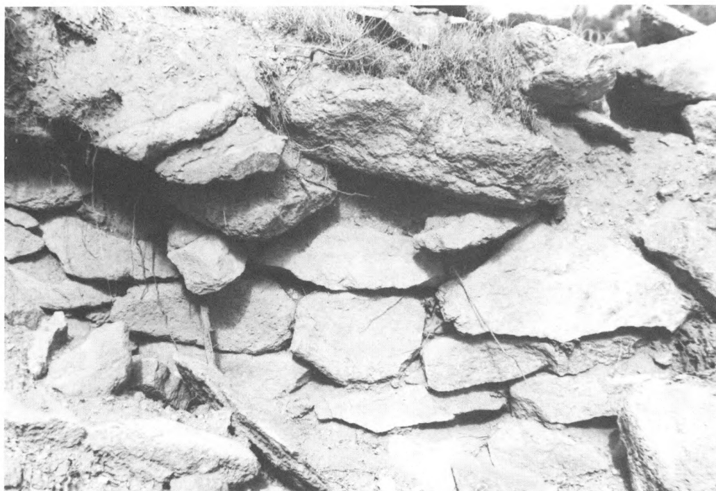
Fig. 8. Wall construction at Site #3.
